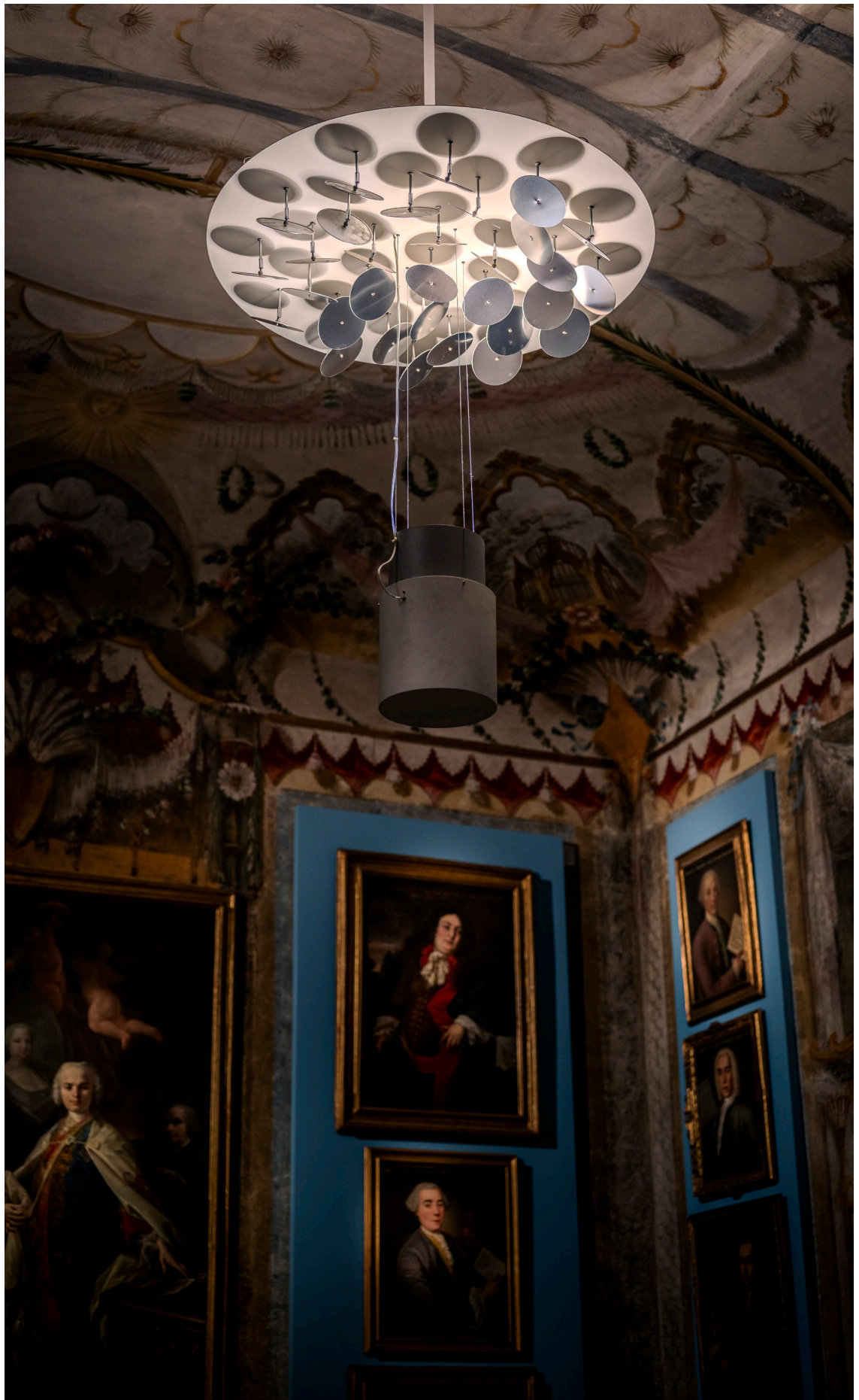
Fig. 01: Detail of the Multireflex light system installed inside the Museo internazionale e biblioteca della musica di Bologna, November 2024. The lighting system takes full advantage of the physical characteristics of the rooms, in particular their height, so that they can be illuminated at 360 degrees without the risk of blinding visitors through glare. Photo by Federico Maria Giorgi.
